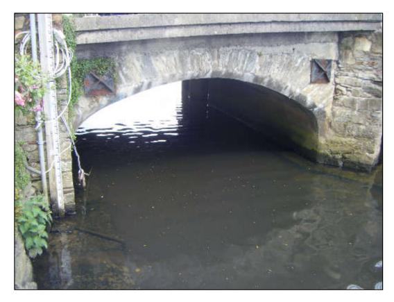
Figure 13 View of the southernmost span of Arklow Bridge (note the concrete encasement around the west abutment)
